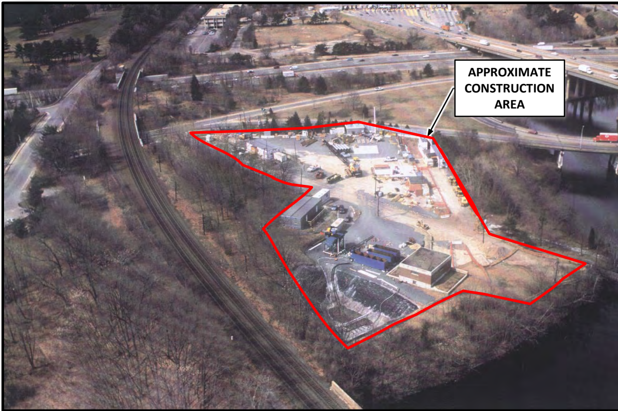
MWWST Shaft 5A – During Construction
